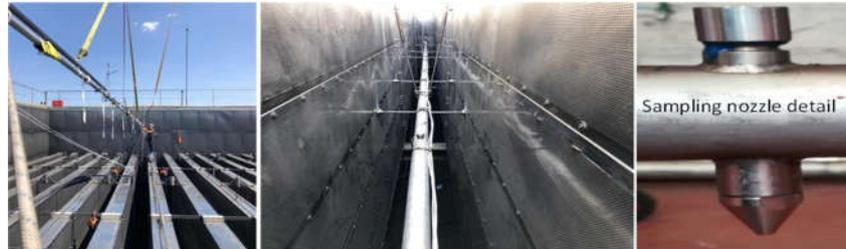
Figure 1. Multi-orifice probe installation at INTA stack (left and centre), and an individual sampling nozzle (right).
